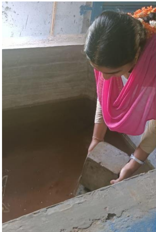
3.12 Curing of concrete
